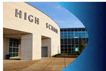
Building with HVAC
