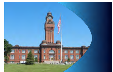
Buildings without HVAC
